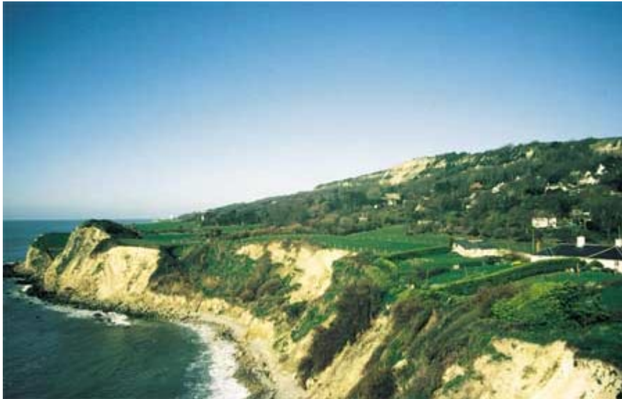
Plate P4a Binnel Point, Ventnor Undercliff Landslide complex, Isle of Wight. Coastal erosion has exposed important palaeo-environmental evidence
